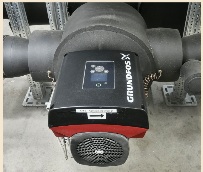
High-efficiency inline pump from the TPE series
