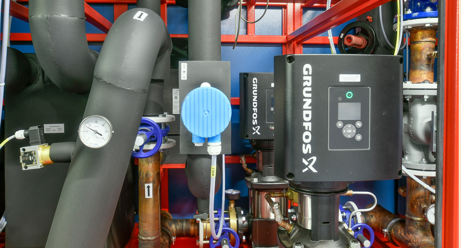
Group of fittings from the high-efficiency SEW heat recovery system
