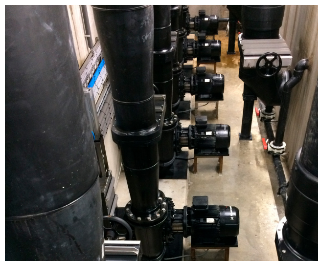
GRUNDFOS pump installation at Kingfish Zeeland
