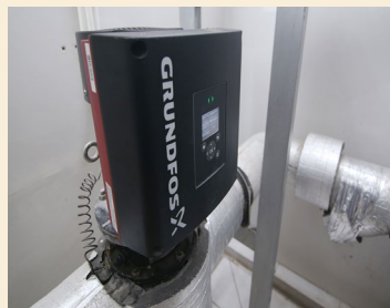
From left to right: MAGNA3 and TPE pumps in Chiller Plant room
