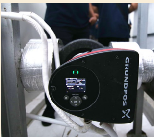
From left to right: MAGNA3 and TPE pumps in Chiller Plant room
