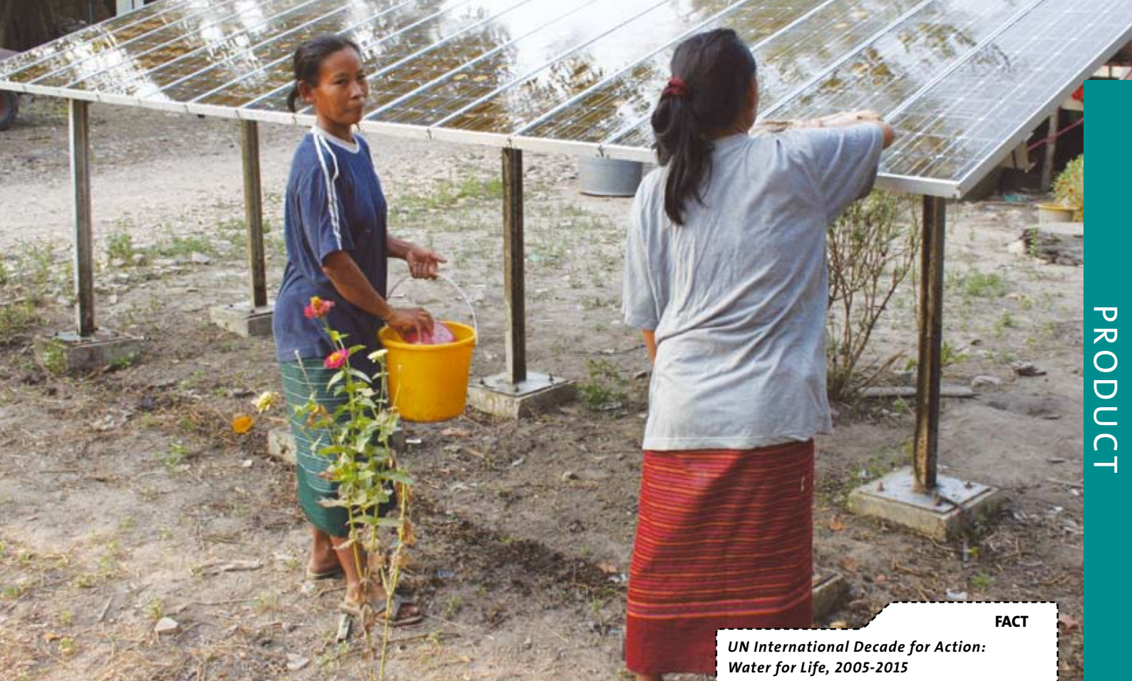
Women in Kudchalert Village cleaning the solar panels used for the SQFlex system.
