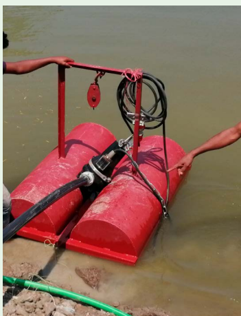
The floating device carrying the submersible pump in the pond
