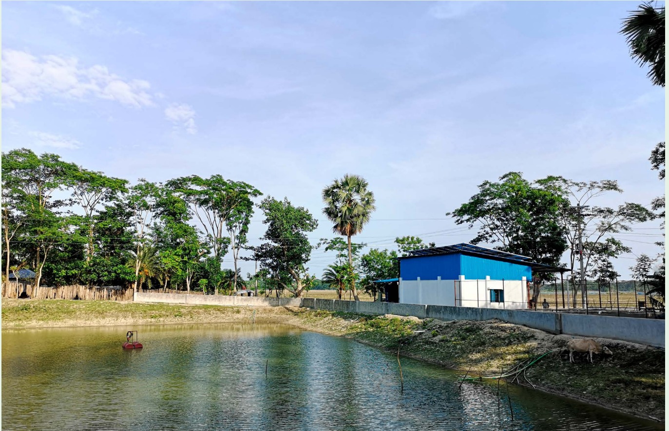
The pond where the submersible pump is installed
