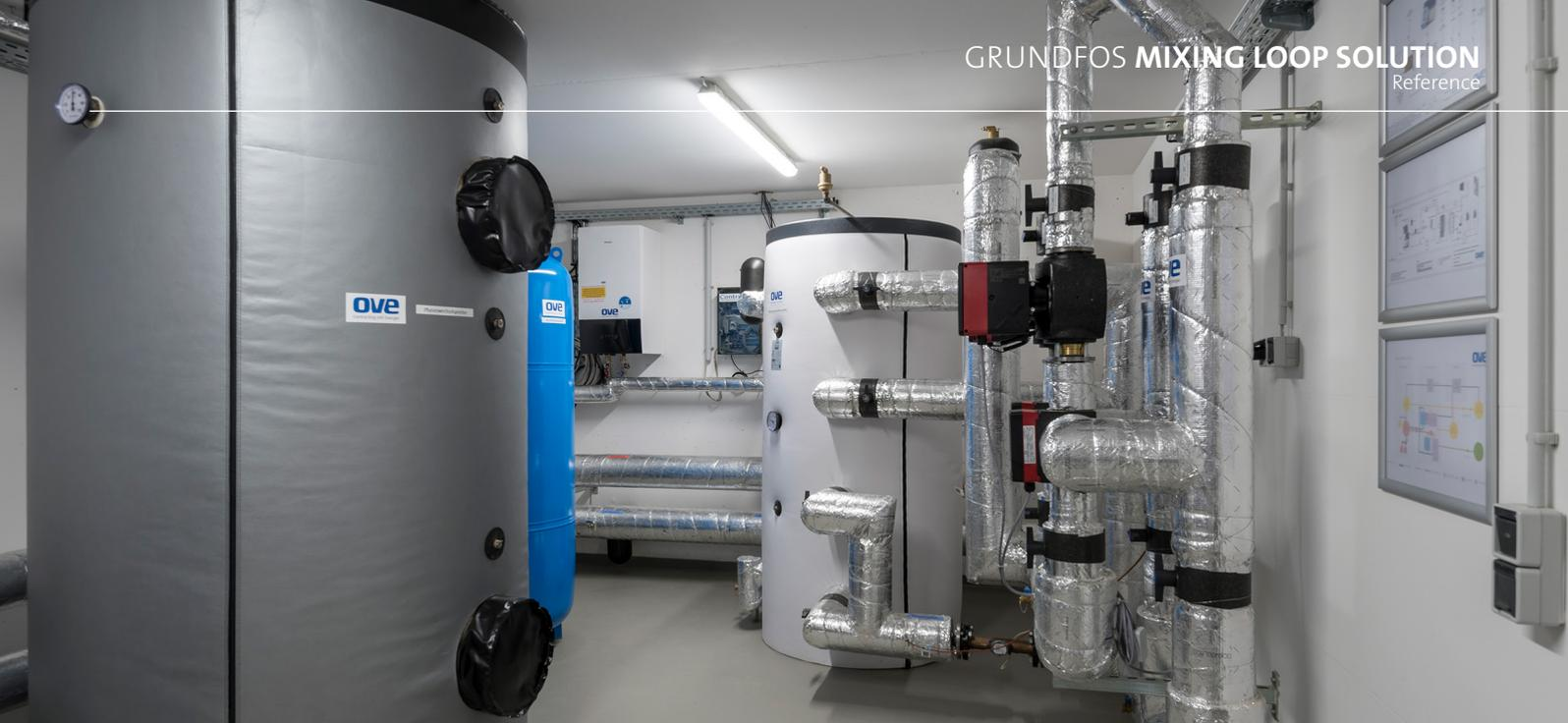
The plant room at the housing estate with phase-change storage CHP system, buffer storage, heat pump and mixing loops
