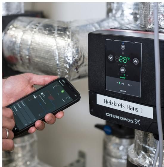
The wireless interface makes it possible to commission and monitor the MIXIT control unit using the Grundfos GO Remote app.
