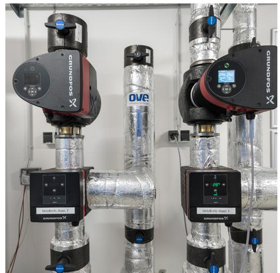
Mixing loops for building phase 1 (right) and 2 (left), each with MIXIT control unit and MAGNA3 secondary circuit pump.
