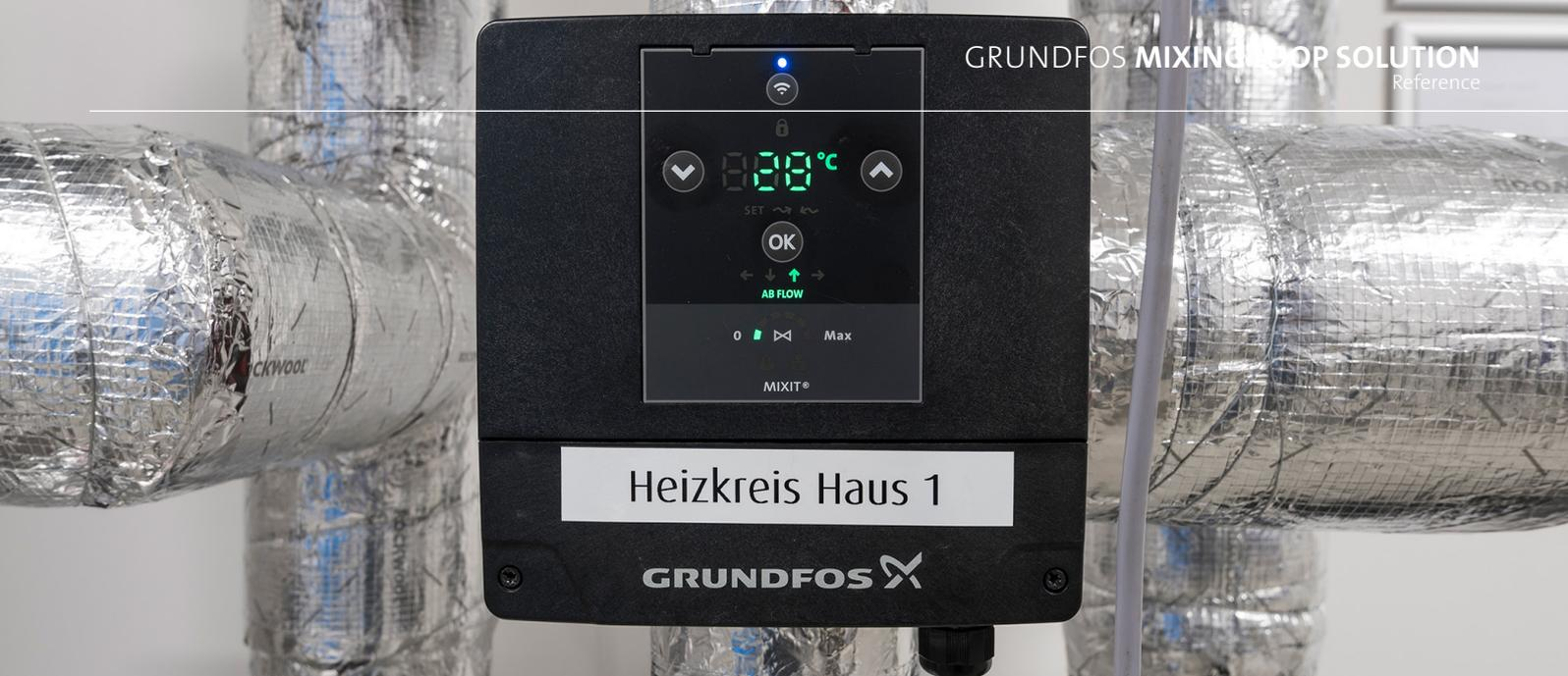
Mixing circuit with MIXIT as 3-way valve: A (bottom) flow from heat generation, B (right) supply circuit return, AB (top) supply circuit flow.
