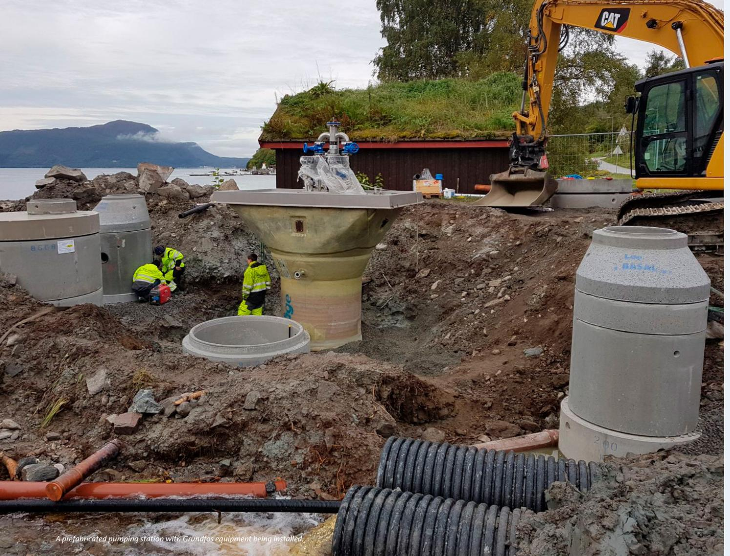
*A prefabricated pumping station with Grundfos equipment being installed.*
