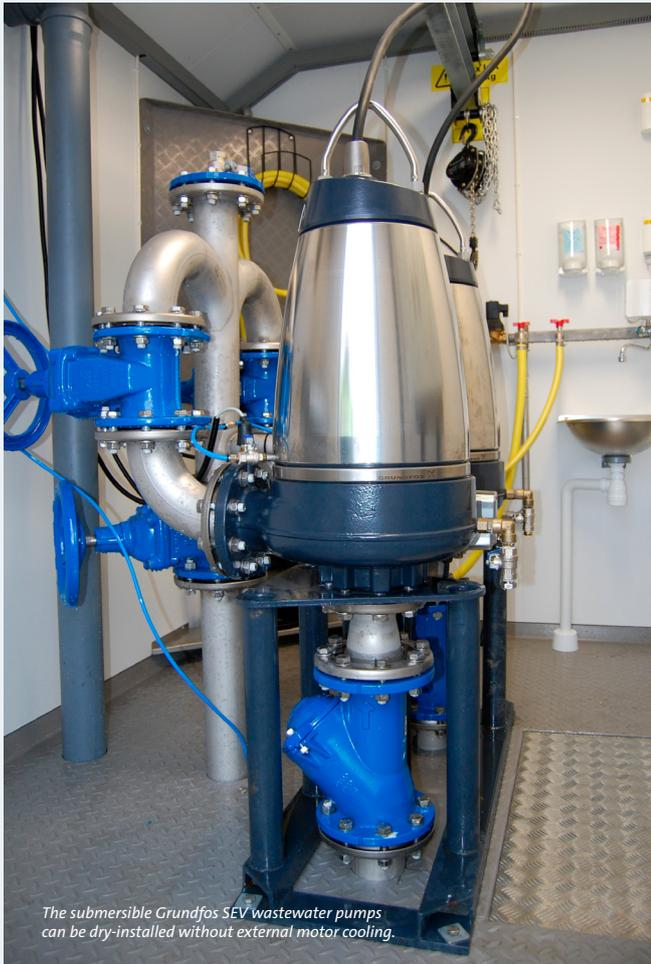
*The submersible Grundfos SEV wastewater pumps can be dry-installed without external motor cooling.*
