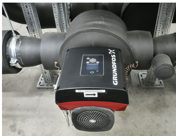
High-efficiency inline pump from the TPE series
