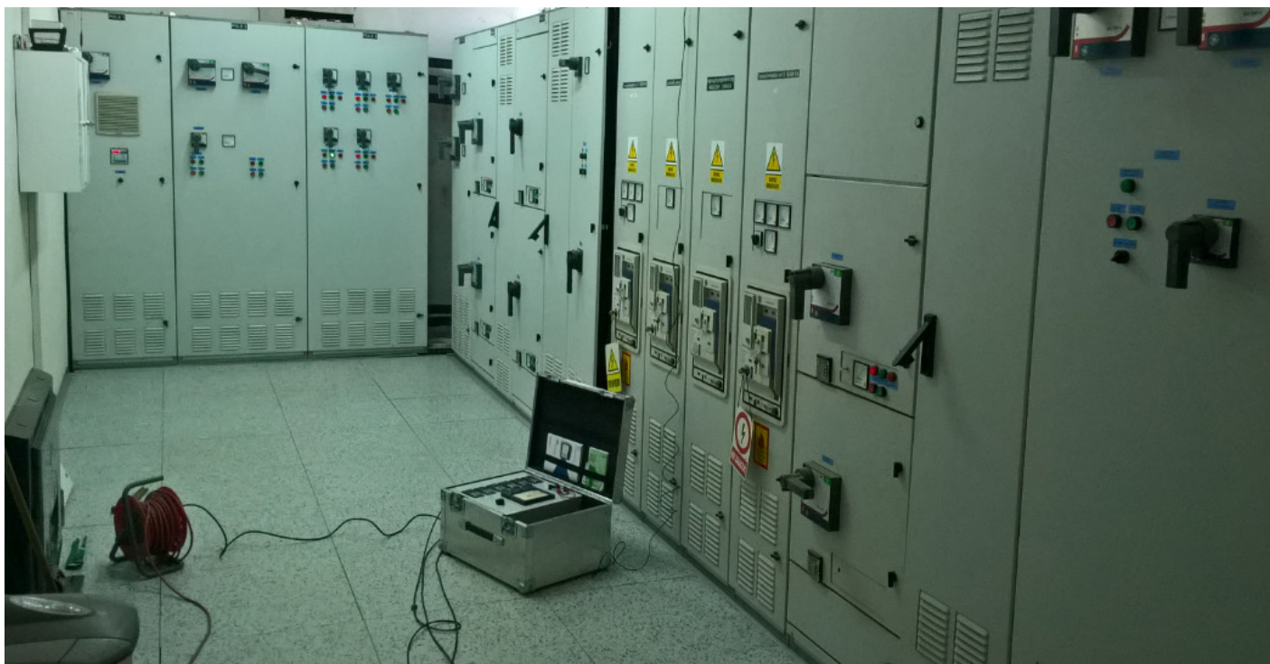
A Grundfos Pump Audit kit is measuring pump system performance in the control room of the Żwirki i Wigury pumping station in Gniezno, Poland.
