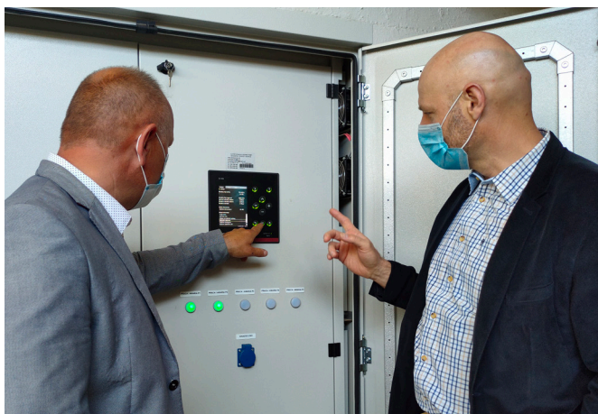
The new Grundfos Control MPC electrical cabinet helped the waterworks manage the city network's water pressure for the best efficiency. It was also integrated into the SCADA system for full overview. Here is Gniezno's Robert Pacanowski with Robert Góra, a Grundfos Sales Engineer.
