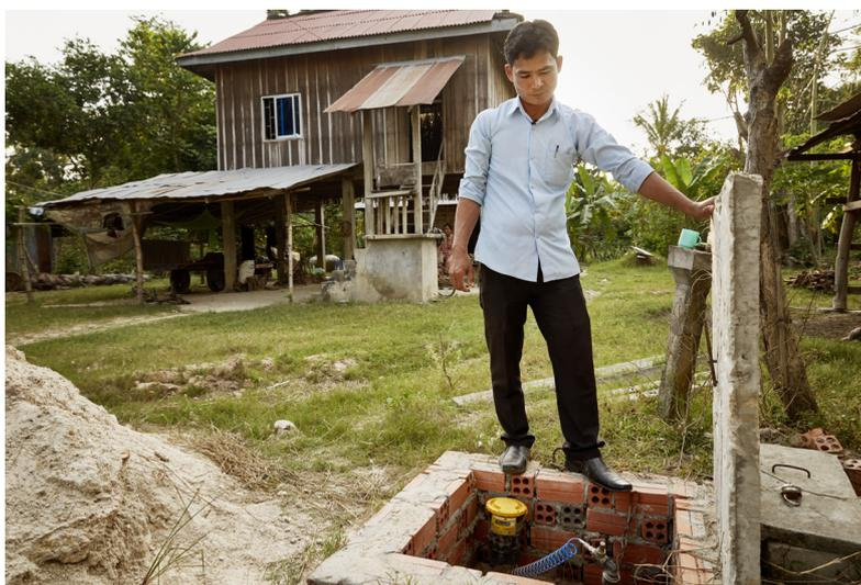
*Em Eang, Head of Supply Network at Takéo Safe Water Supply, inspects the remote sensor at one of the critical points on the water plant's network – in Prek Pha-Aov village, 10 km from the station. The sensor collects daily water consumption data and sends it back to the central controller to automatically adjust the system's load profile.*
