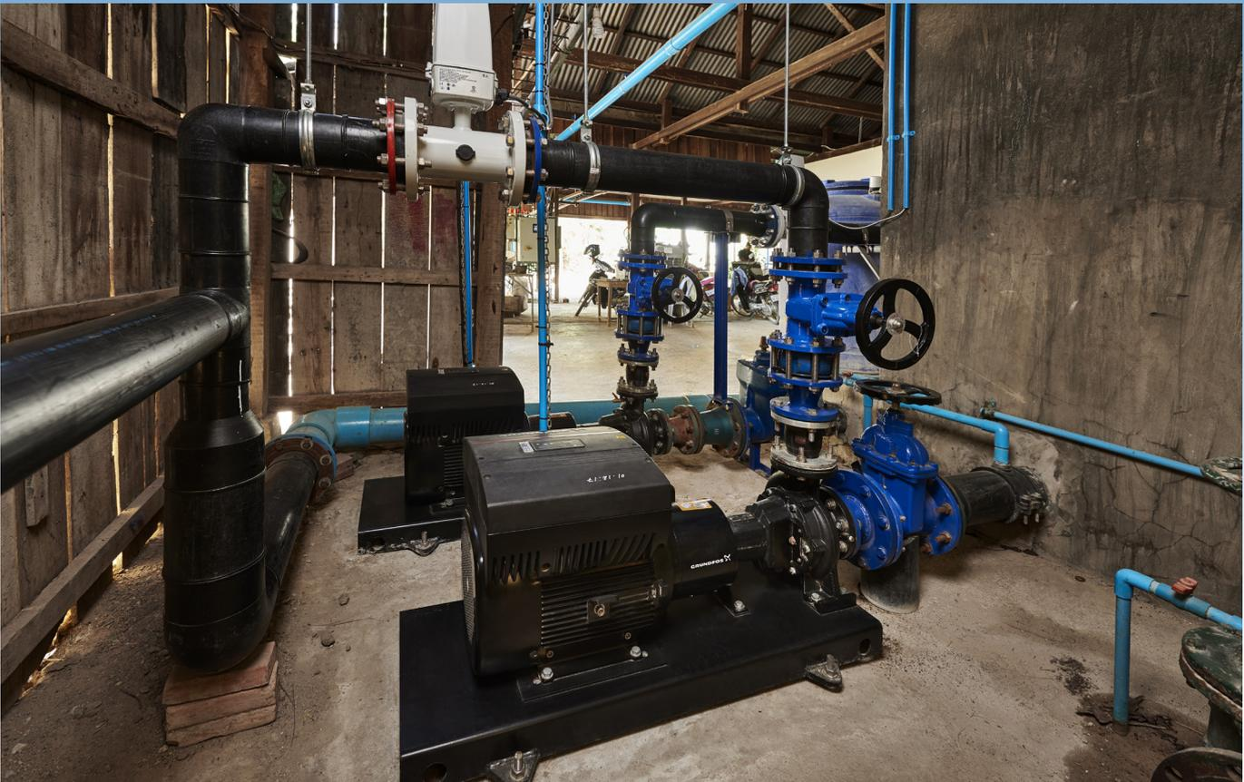
Grundfos NKE pumps are the heart of the Demand-Driven Distribution system at Takéo Safe Water Supply in Cambodia.
