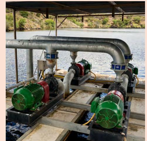
Grundfos NK65-250 end-suction pumps move water from one of the main river reservoirs to a holding dam partway up the farm’s hilly terrain. They operate from a floating structure in the lake.
