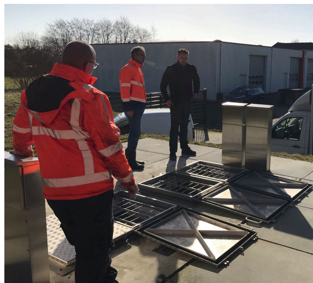
The satisfied Operations Manager, Ivo ten Brinke (right), shows around the new pumping station.
