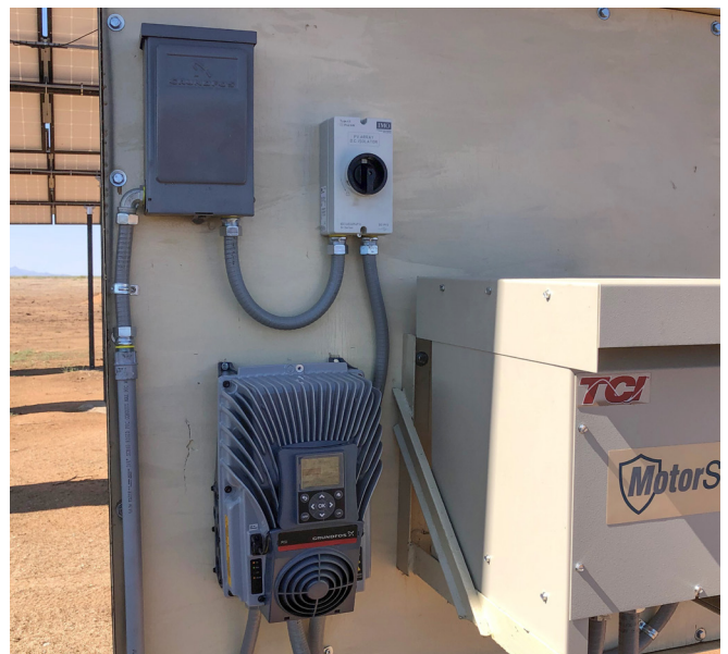
The Grundfos RSI (Renewable Solar Inverter) providing power to the SP pump and motor.
