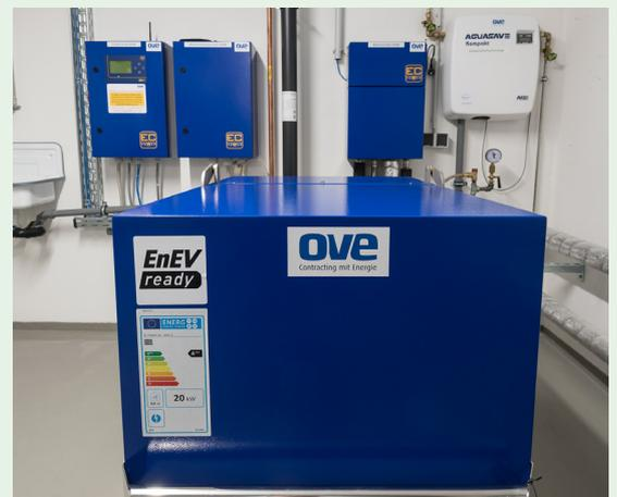
The main heat generator is a compact CHP system with 21 kW of thermal and 9 kW of electrical output.
