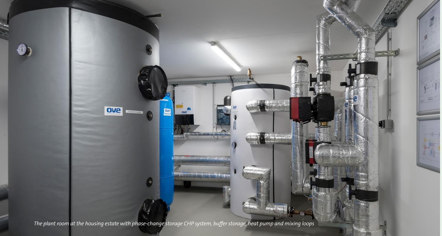
The plant room at the housing estate with phase-change storage CHP system, buffer storage, heat pump and mixing loops
