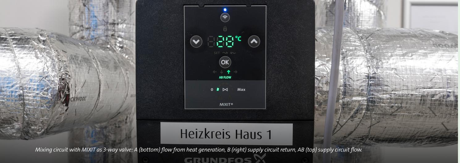
Mixing circuit with MIXIT as 3-way valve: A (bottom) flow from heat generation, B (right) supply circuit return, AB (top) supply circuit flow.
