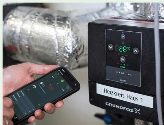
*The wireless interface makes it possible to commission and monitor the MIXIT control unit using the Grundfos GO Remote app.*
