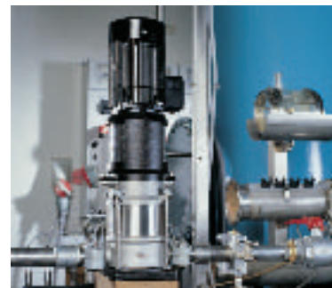
CRN-pump with MAGdrive. The magnetic drive design eliminates the need for shaft sealing. The pump is ideal for heavy-duty industrial applications.
