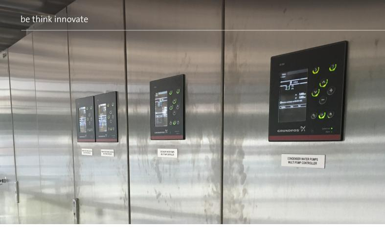
"The Grundfos iSOLUTIONS is a key element in this cider manufacturer's continuous improvement for their cooling system, as it reacts immediately to process or demand changes."
