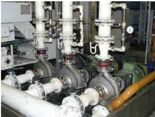
These three MWF pumps were the focus of attention during the Pump Audit pilot project - due to their cost-effectiveness, they will remain in operation.
