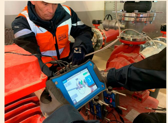
A laser alignment tool helps to make sure the pump motor shaft is in line on the Grundfos fire pumps.
